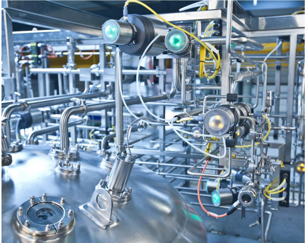
Picture shows intelligent control heads on various sizes of process valve in a pharmaceutical production environment. Using the TopControl Type 8694 from Bürkert allows full valve control using a fieldbus network, reducing the wiring required by decentralizing control.
