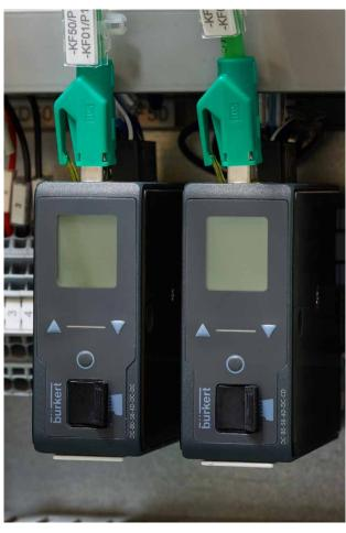
The current flow of all cooling circuits is constantly transmitted to the upstream casting process controller via the Profinet gateway ME43. Downtime can be reduced thanks to reliable process monitoring.
