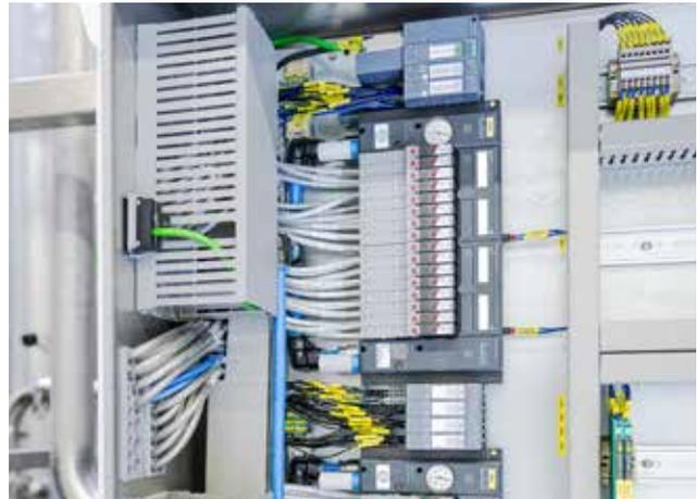
The valve island Type 8647 is designed for installation in control cabinets and can be mounted on standard rails to save space.
